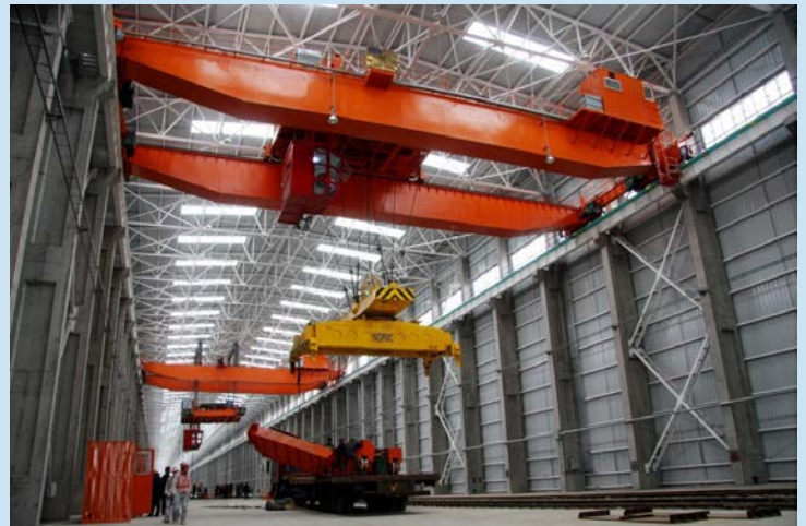
Asia's Largest Rail Inland Trans-loading Centre in Alashankou, Xinjiang, PRC.
